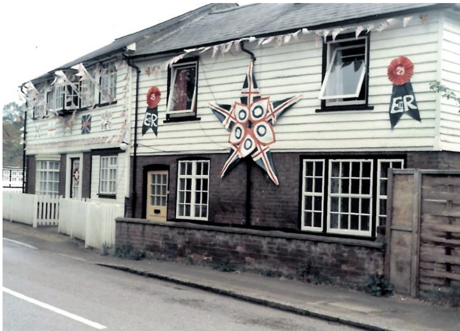
33 Lemsford Village built before 1833
